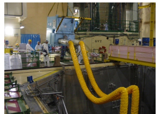
MED CP® installation on a cover tank to apply negative pressure to the primary circuit
